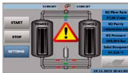
Touch Screen PLC - Pic. 2
